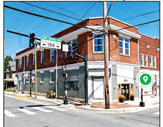
Hesson's Department Store building as it appears today.
