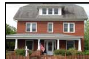
306 East Main St.
